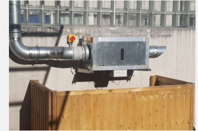
Installing the VMI® system in one section in each nursery
