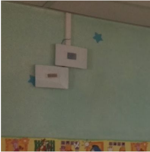
Installing the IAQ monitoring devices (CO 2 , RH, T, TVOC, PM)
